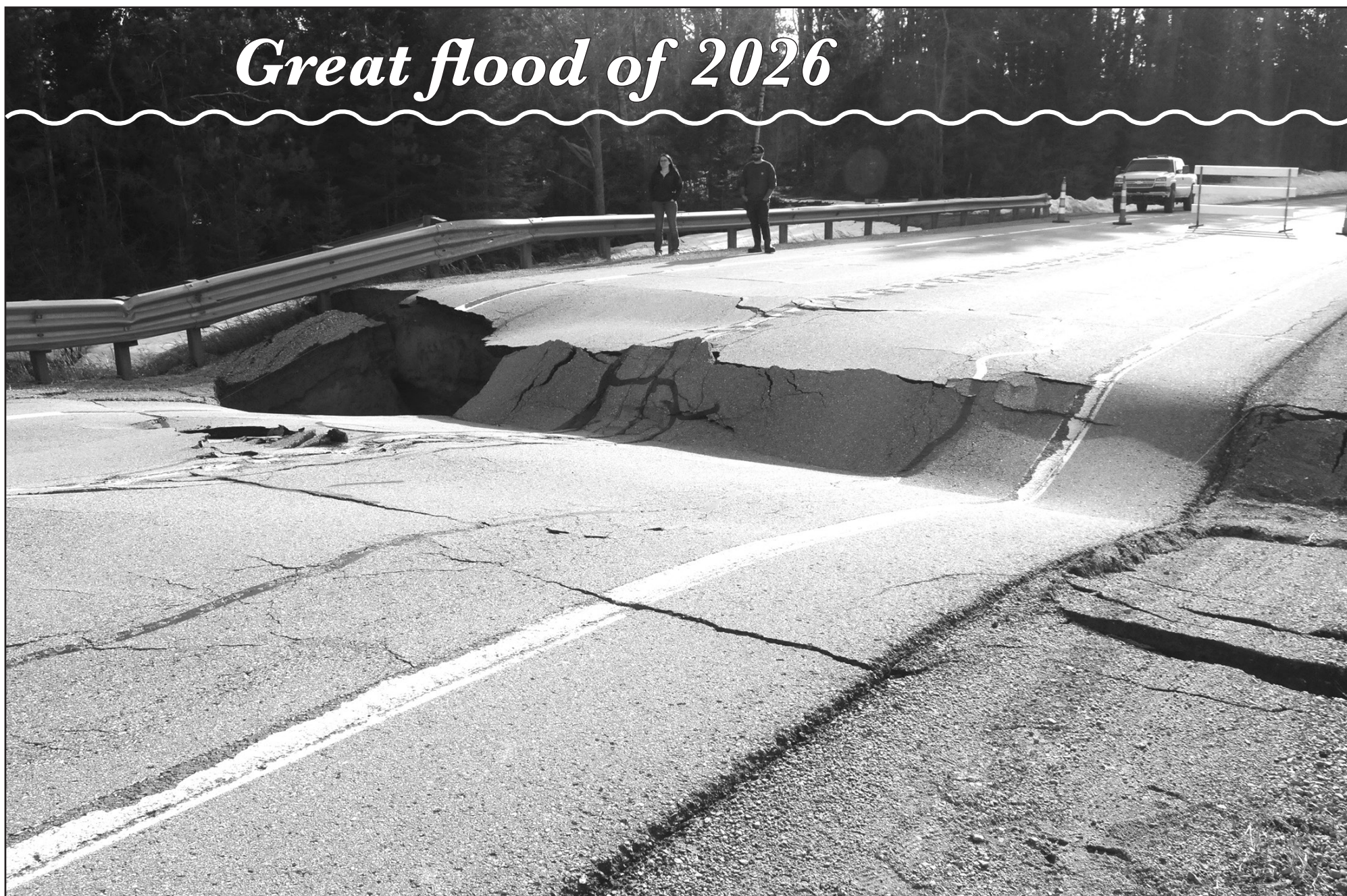
A washed out M-68 (top) will require several weeks to repair after suffering major damage.
