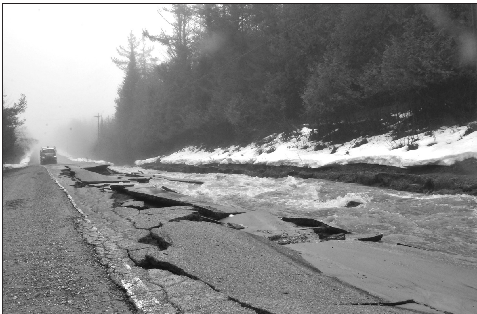
A washed out M-68 (top) will require several weeks to repair after suffering major damage.
