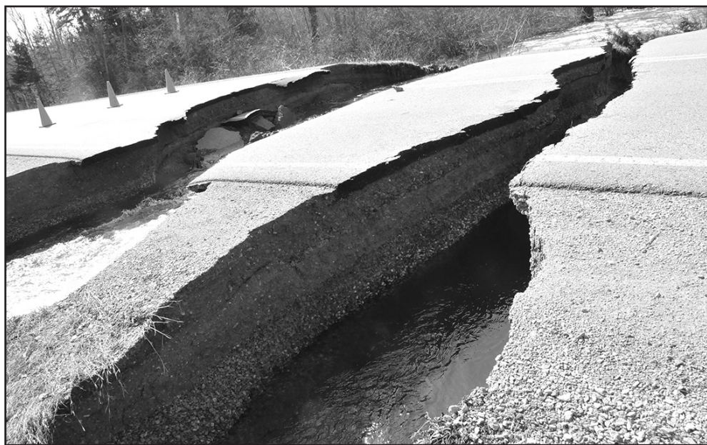
County Road 451 is closed south of Heythaler Highway after floodwaters ripped through the roadway.
